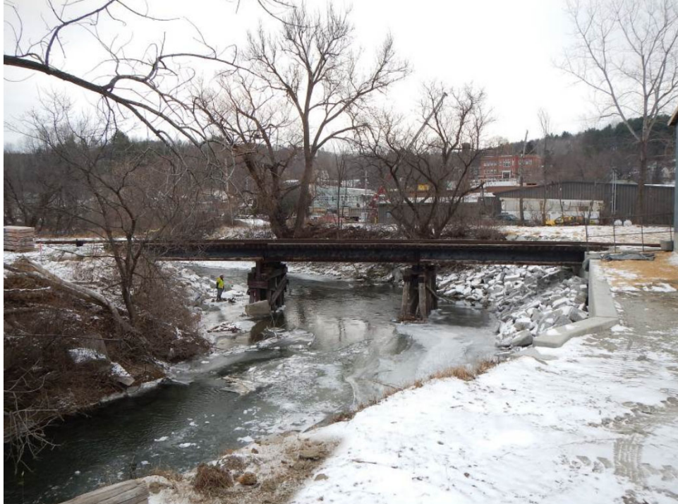
Looking downstream along Stevens Branch at Bridge 308
