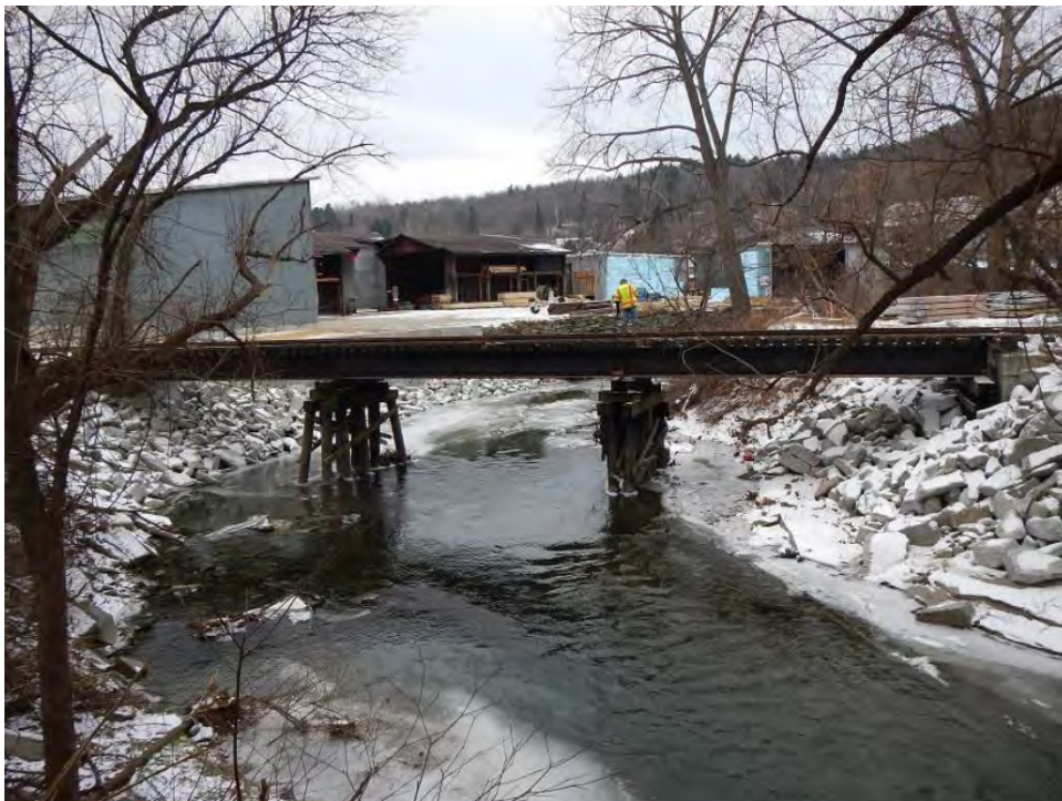
Looking upstream along Stevens Branch at Bridge 308
