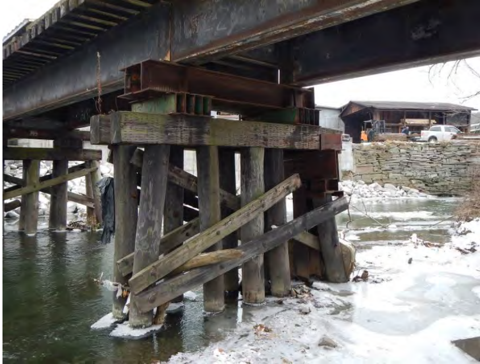
Looking at Pier 1 from west bank
