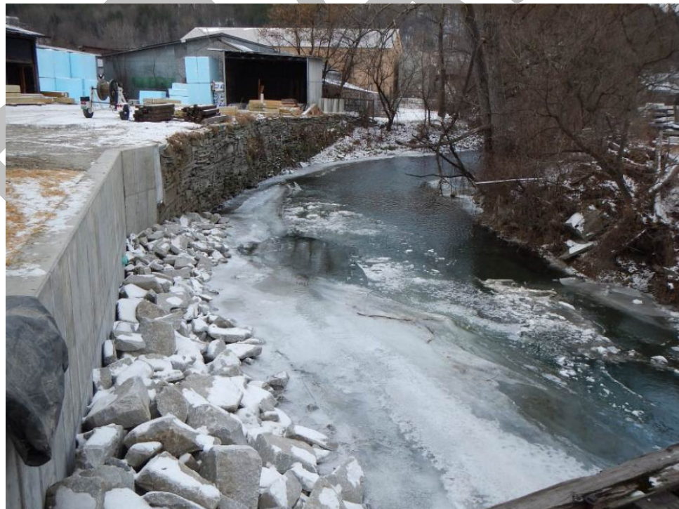
Looking upstream at Stevens Branch from Bridge 308
