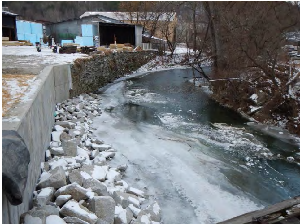
Looking upstream at Stevens Branch from Bridge 308
